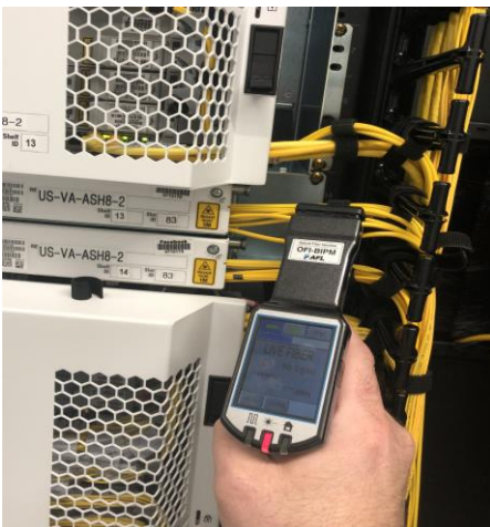
Figure 1 : Active in-use fiber detection on a line side DWDM system fiber. Image supplied by Meta
